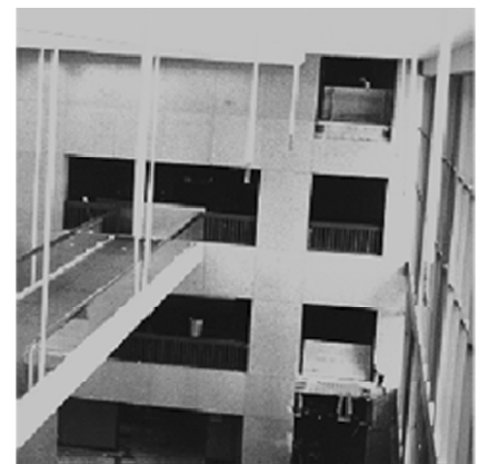
Figure 1 - Third Floor Walkway (left)
