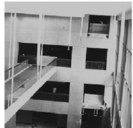
Figure 1 - Third Floor Walkway (left)
