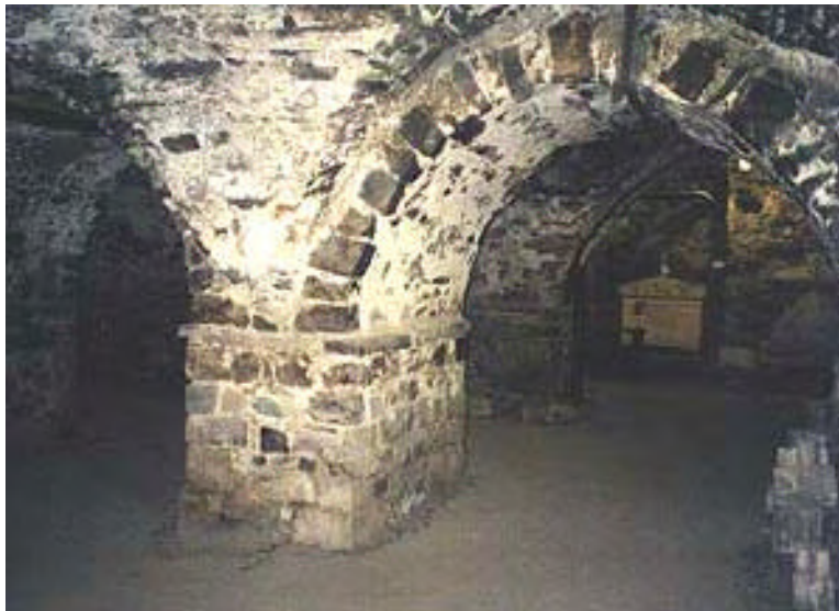
Photograph 1.1 - Foundations for a Medieval Era Cathedral
