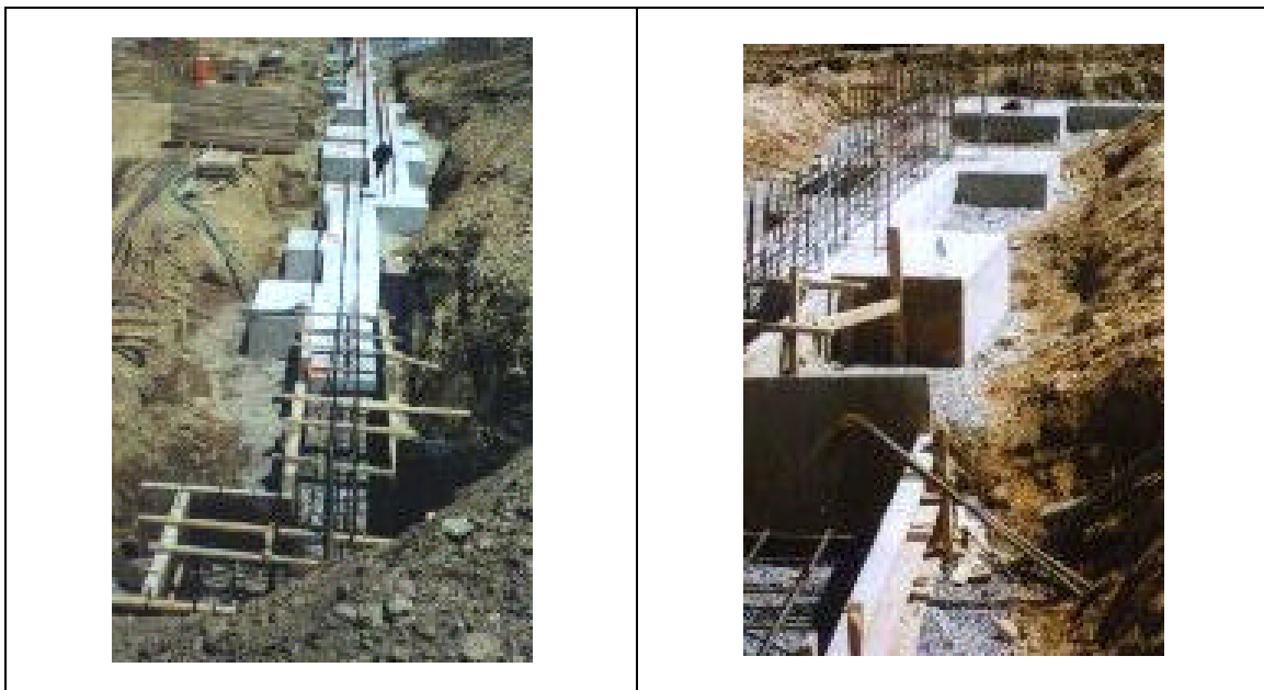
Photograph 4.1 – Shallow Spread Footings
