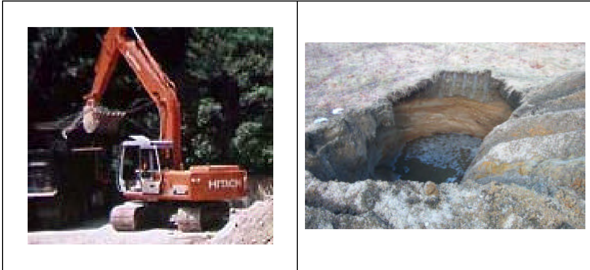
Photograph 2.1 – Test Pit Excavation
