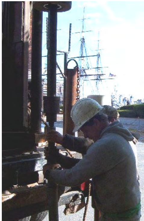
Photograph 2.2 – Standard Penetration Test
